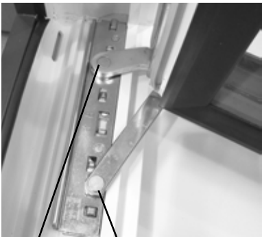
1 2 Corner bearing bottom
