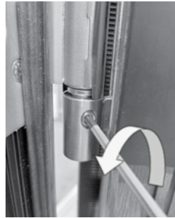
Loosen fixing screw.
